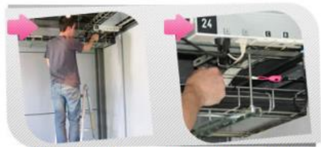
pulling out cables for passage in false ceiling or cable tray
